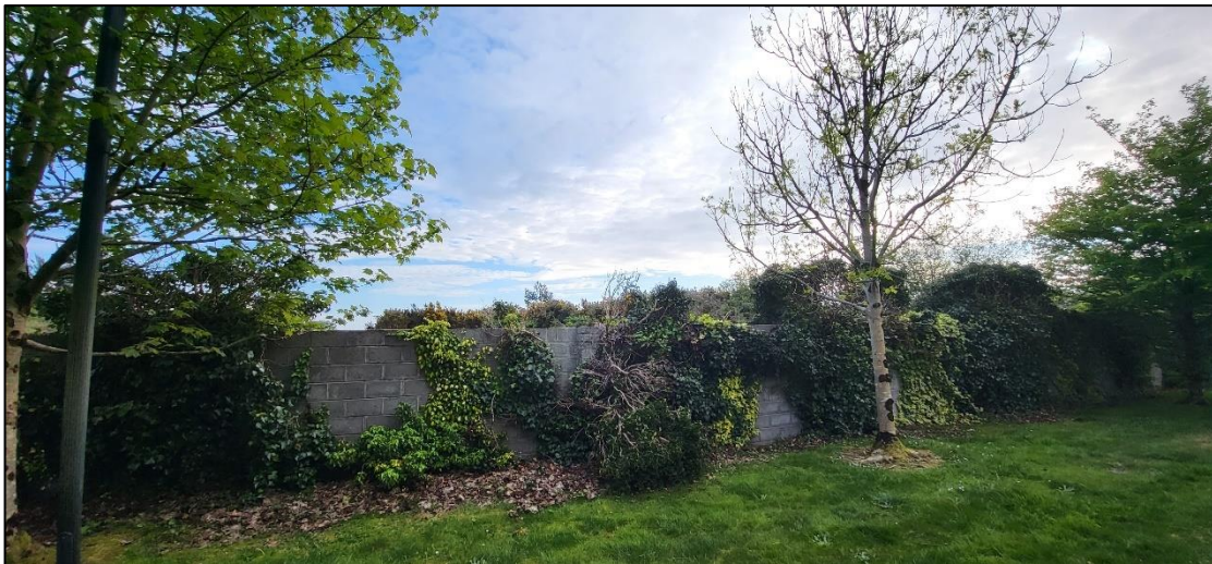
Plate 13-17 View towards the Proposed Development from the Back of An Logan Housing Estate
