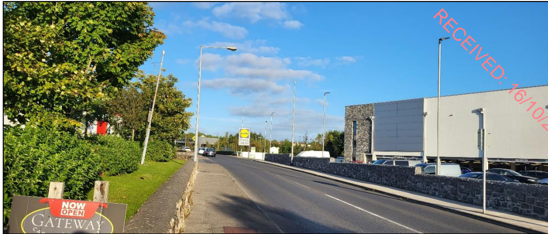
Plate 13-11 Retail and Commercial Buildings to the North of the Proposed Development site
